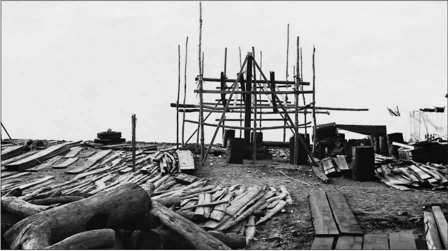
The early stages of construction – setting up the stem and the sternposts (photo courtesy of Rainer Hartel)
